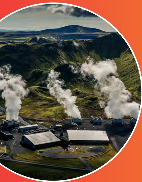
Climeworks has a direct air carbon capture plant in Iceland.
